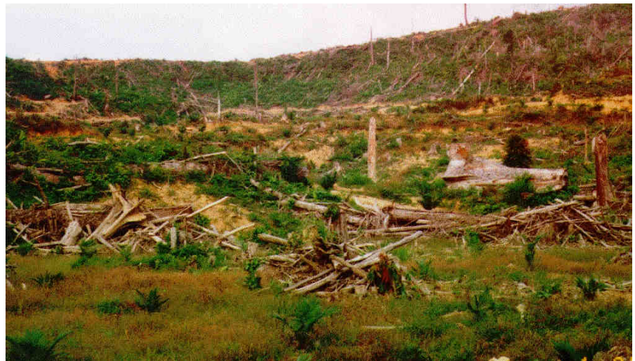
Plate 4.9: Vegetative wastes from site clearing may be left on site (preferably properly stacked) to degrade naturally instead of being burnt
