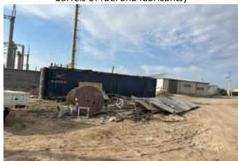
Lack of designated storage for construction waste: debris and used construction materials were piled near the technical trailer and partly outside the construction site
