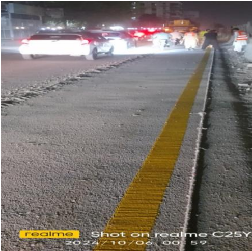
Lane Marking at Sheikh Zayed
