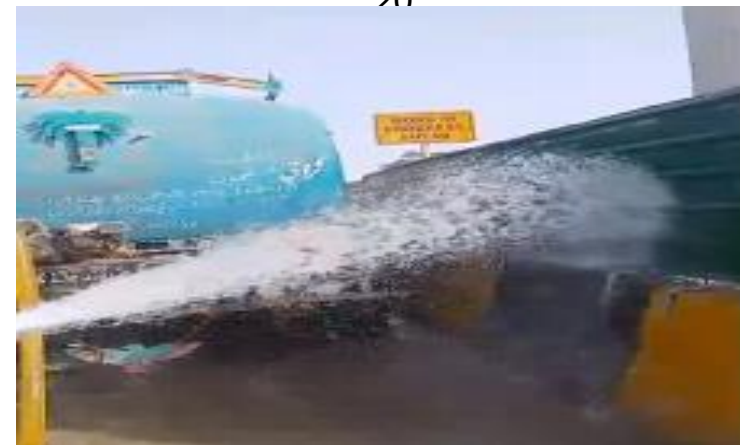
Washing of NJ barriers and Fence from (Karachi University to Shaikh Zayed)
