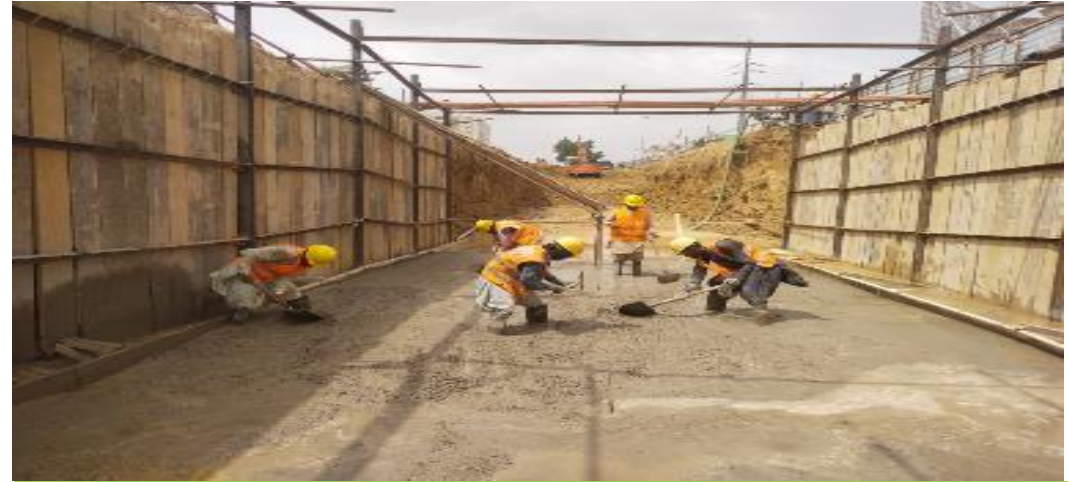
Shoring Work DC-2 at Mosamiyat
