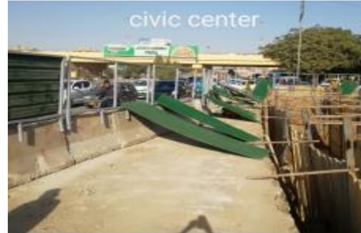
Installation of fiber fence on N.J Barrier at DC-20
