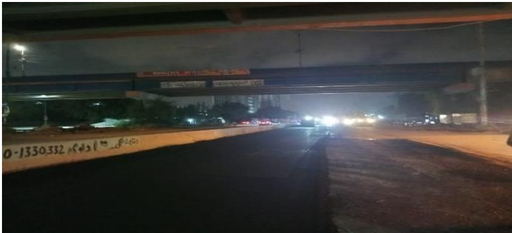
Asphalt Patch Work at NIPA
