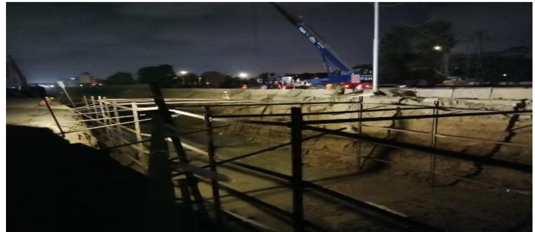
Fixing of Shoring at DC-12 Hassan Square
