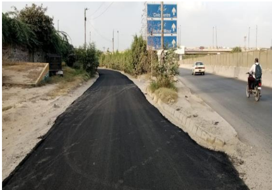
Road patch Work at Safari Park Ramp for smooth traffic flow
