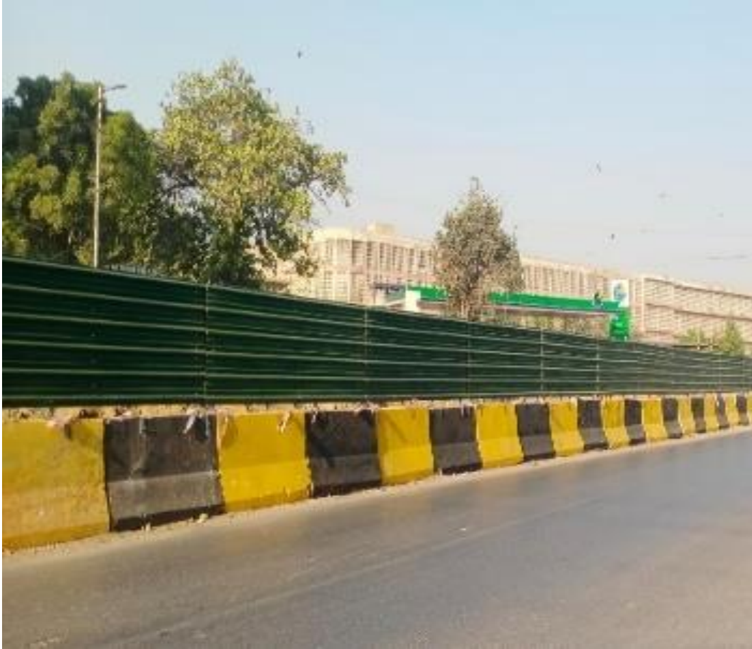
Fiber Fence on N.J Barrier at DC-19
