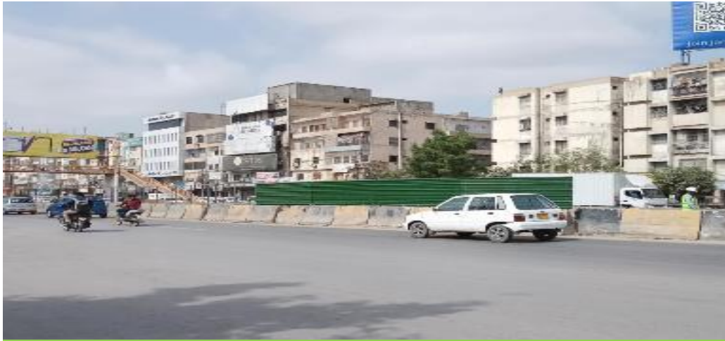
Fiber sheets on NJ Barriers Near Urdu University
