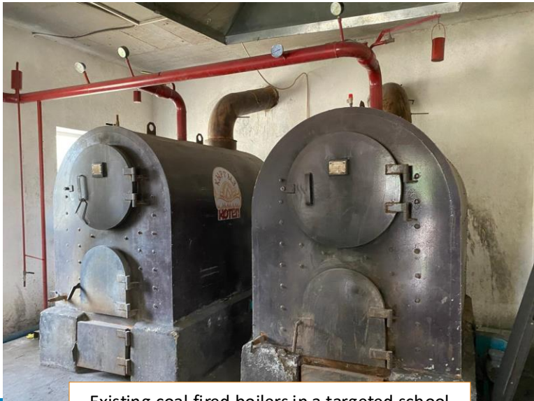
Existing coal-fired boilers in a targeted school
