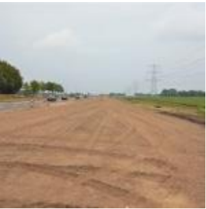
Building waste granulate for road foundation (downcycling)
