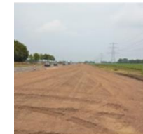
Building waste granulate for road foundation (downcycling)
