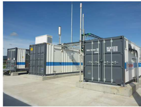
Rectifier/ Electrolyzer/ Gas Compressor
