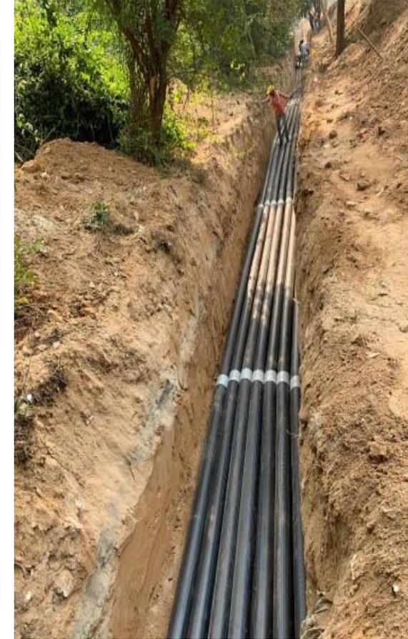
**Laying of 11 kv U/G Cable at Manesar**
