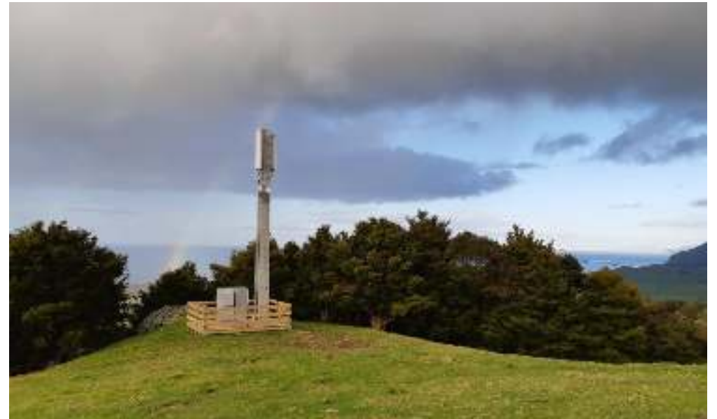
Three-carrier RAN sharing tower in rural New Zealand
