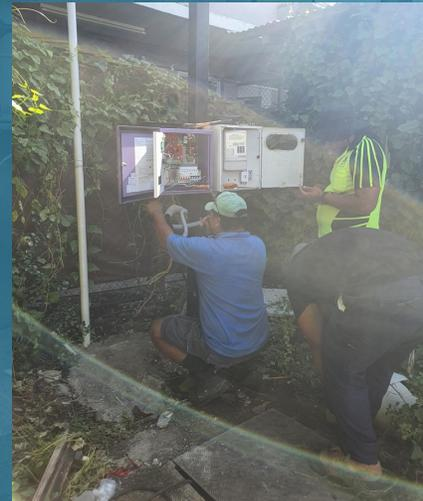
SWA team installing smart control panel for better flow controls and data logging
