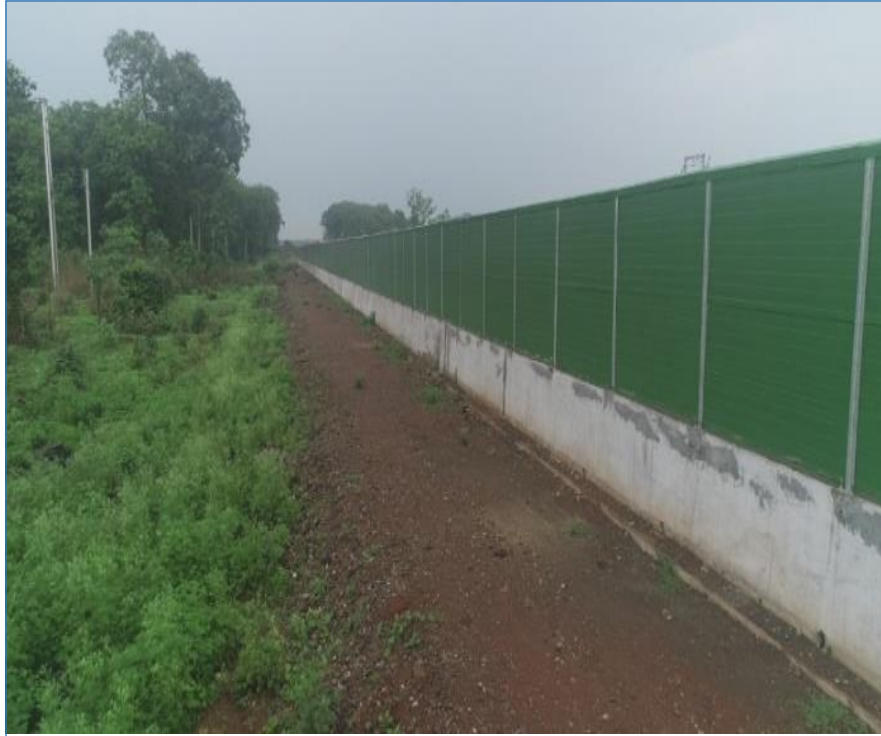
Sound and Noise barrier installations on animal crossings in Pench National Park, Madhya Pradesh
