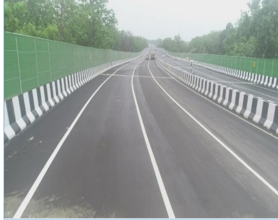
Sound and Noise barrier installations on animal crossings in Pench National Park, Madhya Pradesh
