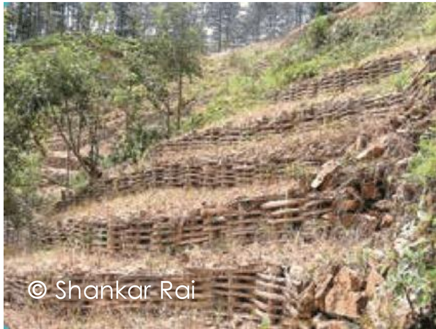
Wattle fence and crib wall
