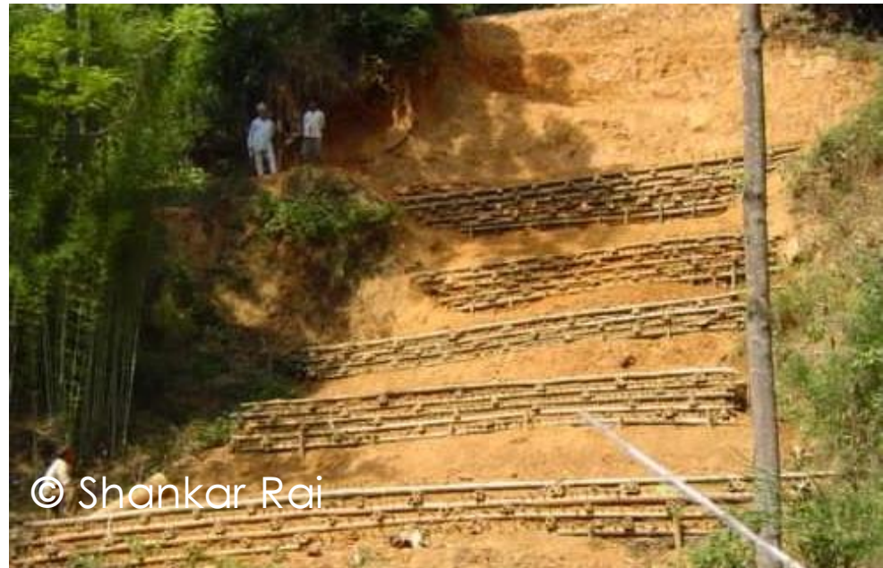
Wattle fence and crib wall
