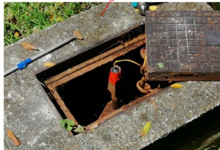
Installed sensor at another washout valve located approximately 160m away.
