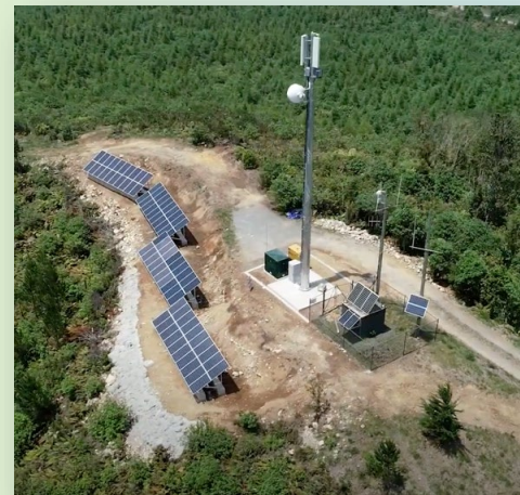
Shared rural LTE tower has three sectors and one microwave backhaul link. Supporting it requires a large solar array plus a diesel generator. Energy requirements take up more than 100 m 2 of land. Source: Photo from Chris Parker. RCG at TECT Park Cell Tower, 2021.
