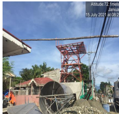
Installation of overhead tank railings and platform at the RHF Photo: PRRM
