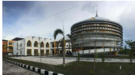
Palangkaraya State Islamic Institute, Bldg. A and Bldg. B, East Kalimantan
