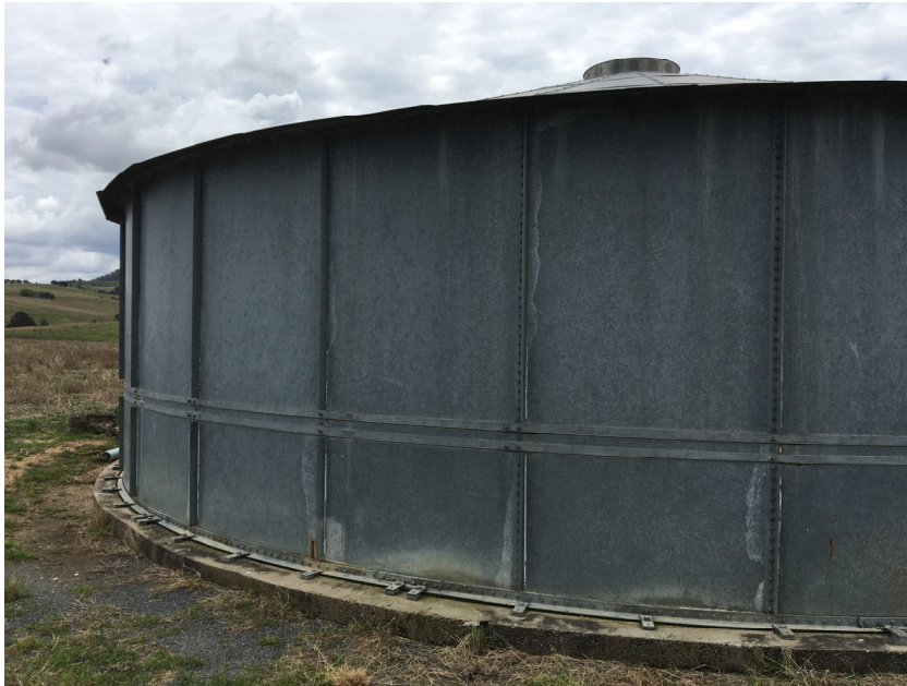
Reservoir: Condition 5 – Evidence of leakage
