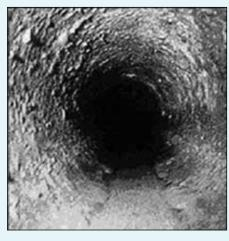
Pipe sediment buildup progressively constricts flow and reduces service.
