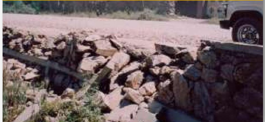
Poor workmanship of a retaining wall, causing collapse – lack of mortar
