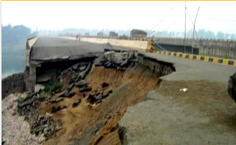
Washed-out approach of bridge
