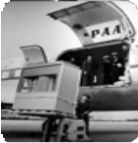
The IBM Model 350 disk file a storage space of 5MB from 1956
