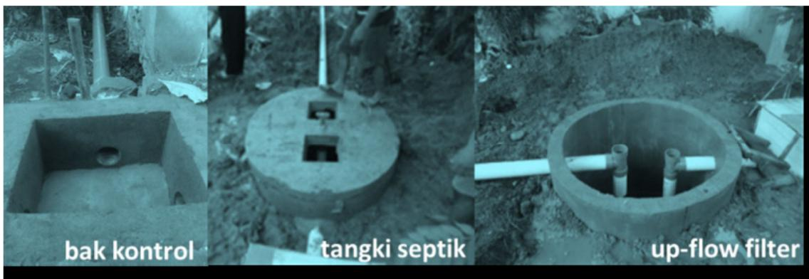
**Installation of Control Box, Septic Tank and Up-Flow Filter** (Source: Ibidem)
