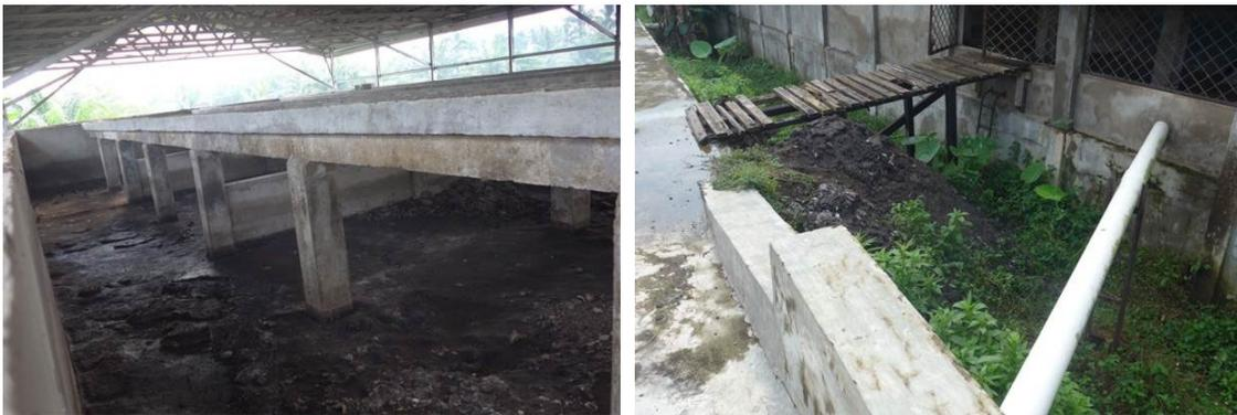
*Figure 36: Sludge Drying Beds*
