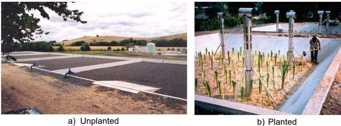
*Figure 53: Sludge Drying Beds*
