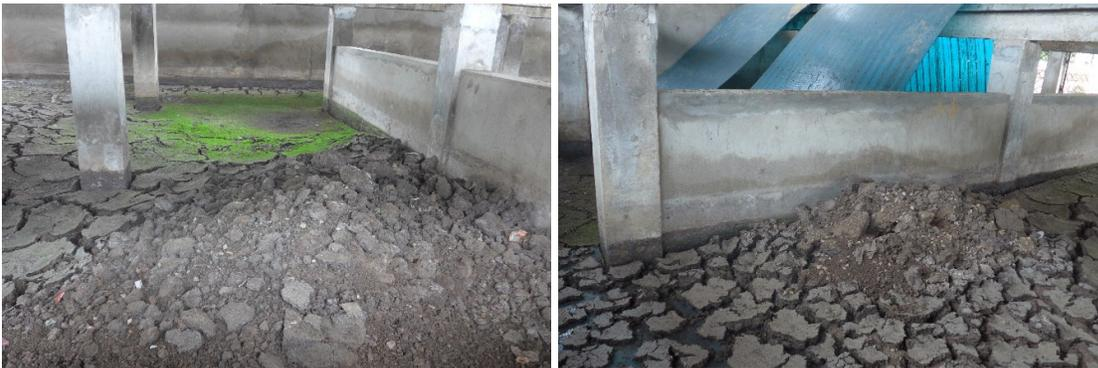
*Figure 52: Dry Sludge Accumulated in the Sludge Drying Beds at the Talang Bakung IPLT*
