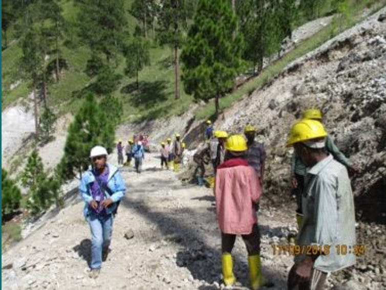
Labour intensive mass balance method Nepal – far less erosion
