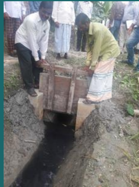
Gated culverts for water management
