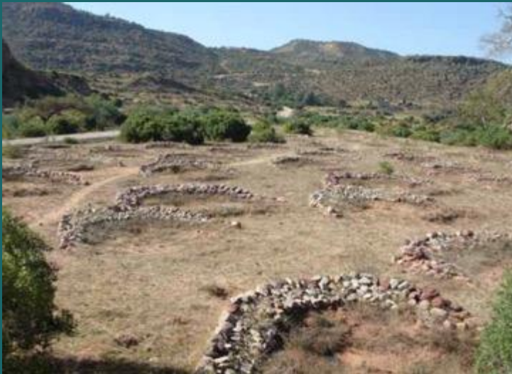
Re-using road material for recharge structures
