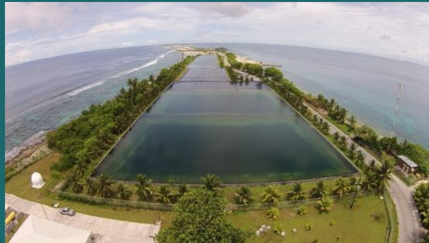
Borrow pits converted to recharge 'water factory'
