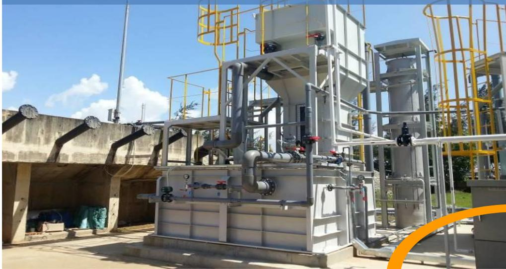
High-rate Trickling Filter (HTF)
