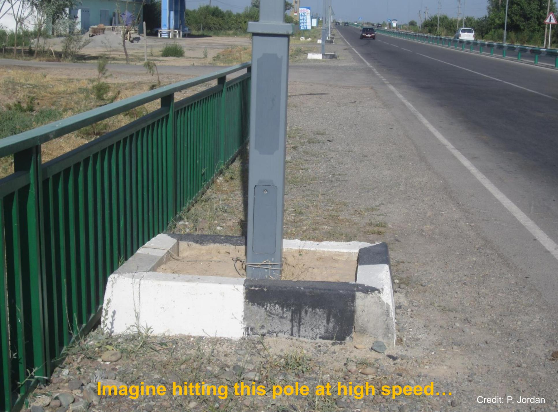
**Imagine hitting this pole at high speed...**
