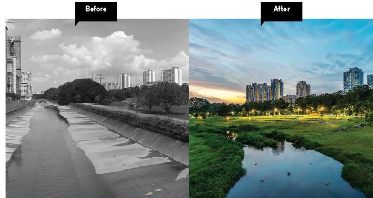
Figure 15. From concrete channel to naturalized river
