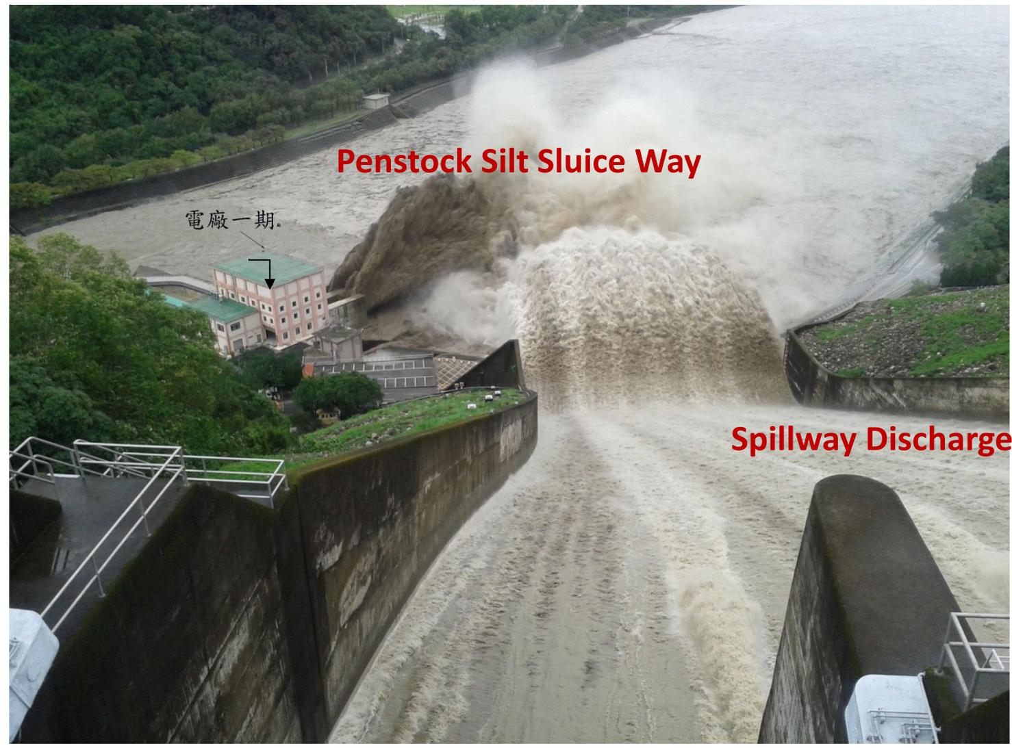
**Penstock Silt Sluice Way**
