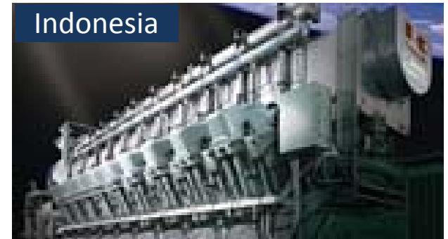
Gas Engine Co-generation system at the automobile assembly plant
