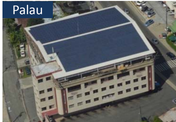
Solar PV installation on the building roof top
