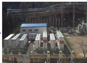
8MW 4MWh Li-Ion Battery in Honam Generators
