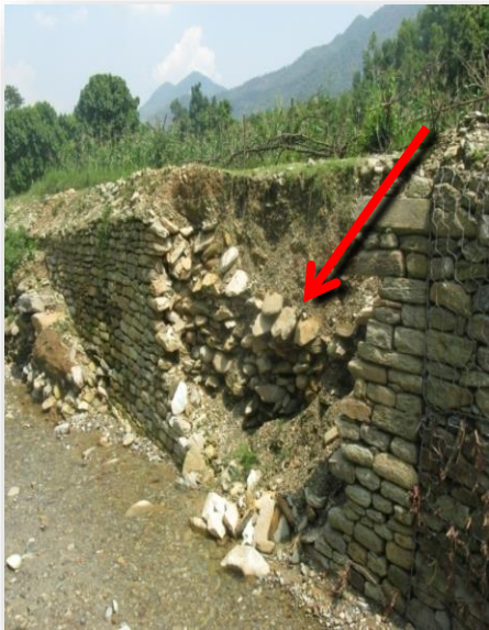
Defective work on gabion boxes
