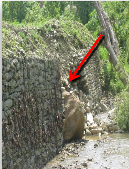
Defective work on gabion boxes
