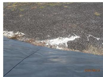
The geotextile protective layer is also destroyed within the active cell as shown below where there are only ribbons of geotextile remaining along the liner batter.
