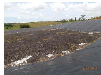
No physical damage of the HDPE liner either within the active or the future cell could be observed. However there may be damage to the liner underneath waste that has been placed previously.
