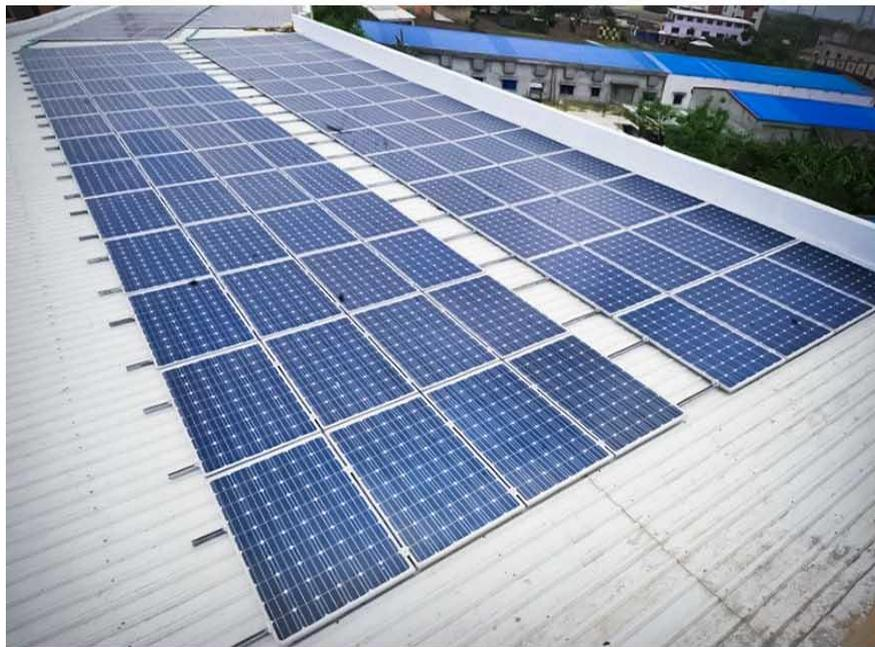
A 65 KW capacity solar power plant with highly efficient mono crystalline panels has been installed in this factory. It will produce at least 110 mw/ hour energy every year which will meet at least 13% of total power required.
