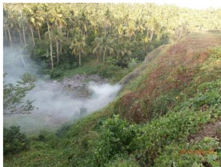
Soil coverage was only partial and extensive areas of insufficient cover were observed. The main batter is at the angle of repose and stable application of final cover soil will not be possible at such steep slopes.
