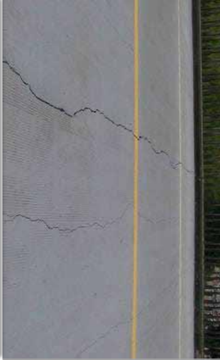
Transverse cracking
