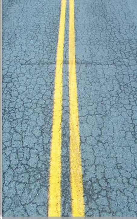
Fatigue cracking
