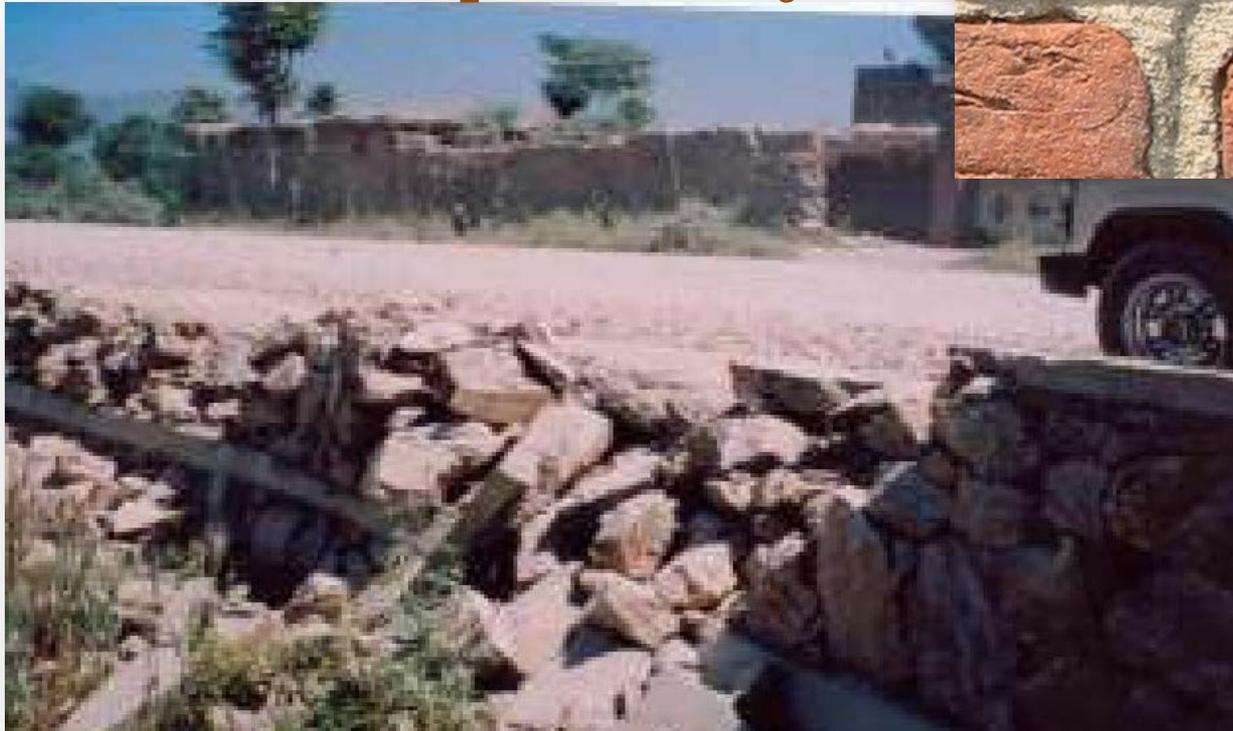
**Poor workmanship of a retaining wall, causing collapse – lack of mortar**
