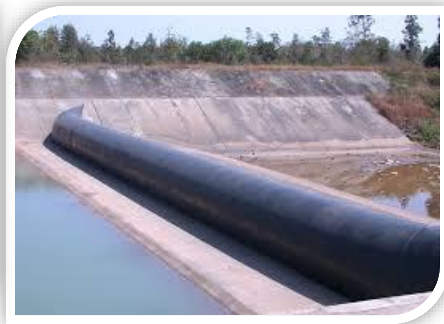
PRC: Inland Waterway Rubber Dam to maintain water level (photo for illustrative purpose)
