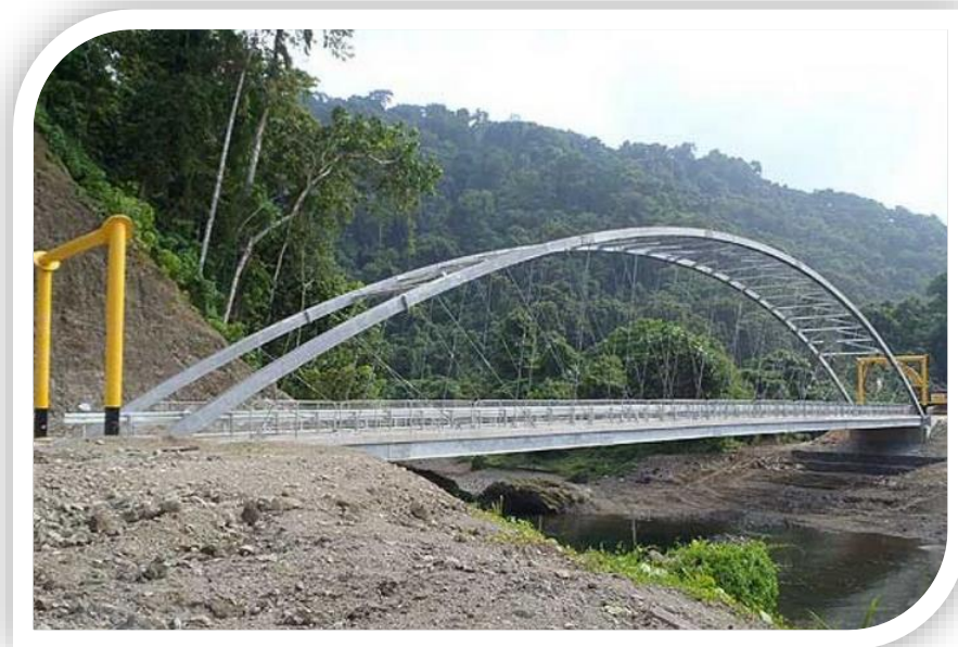
Bridge constructed for higher flood and river debris load
