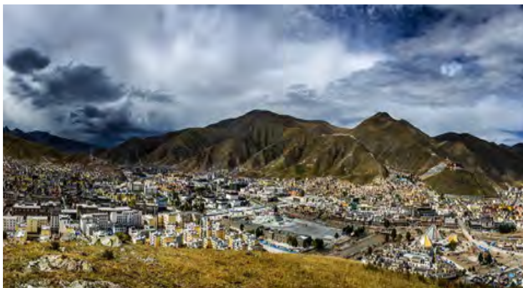
青海玉树州(地震前)/Yu Shu City (Before Earthquake 2010)
