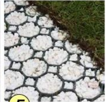
Open-Celled Paving Grid with Gravel
