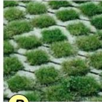
Open-Celled Paving Grid with Vegetation
