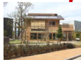
Eco House FC: 1kW × 1units
