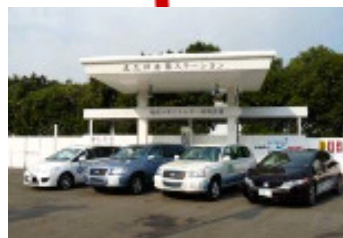
Kitakyushu Hydrogen Station FC: 3kW × 1unit
