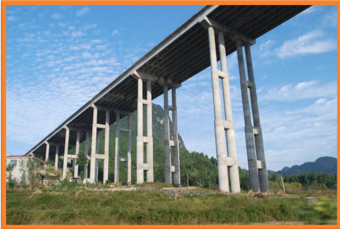
Bridge work in China
