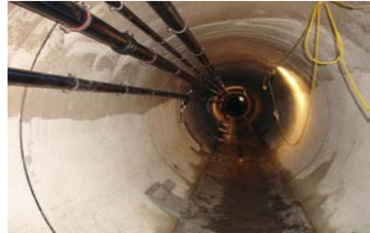
Heat exchanger in sewers
