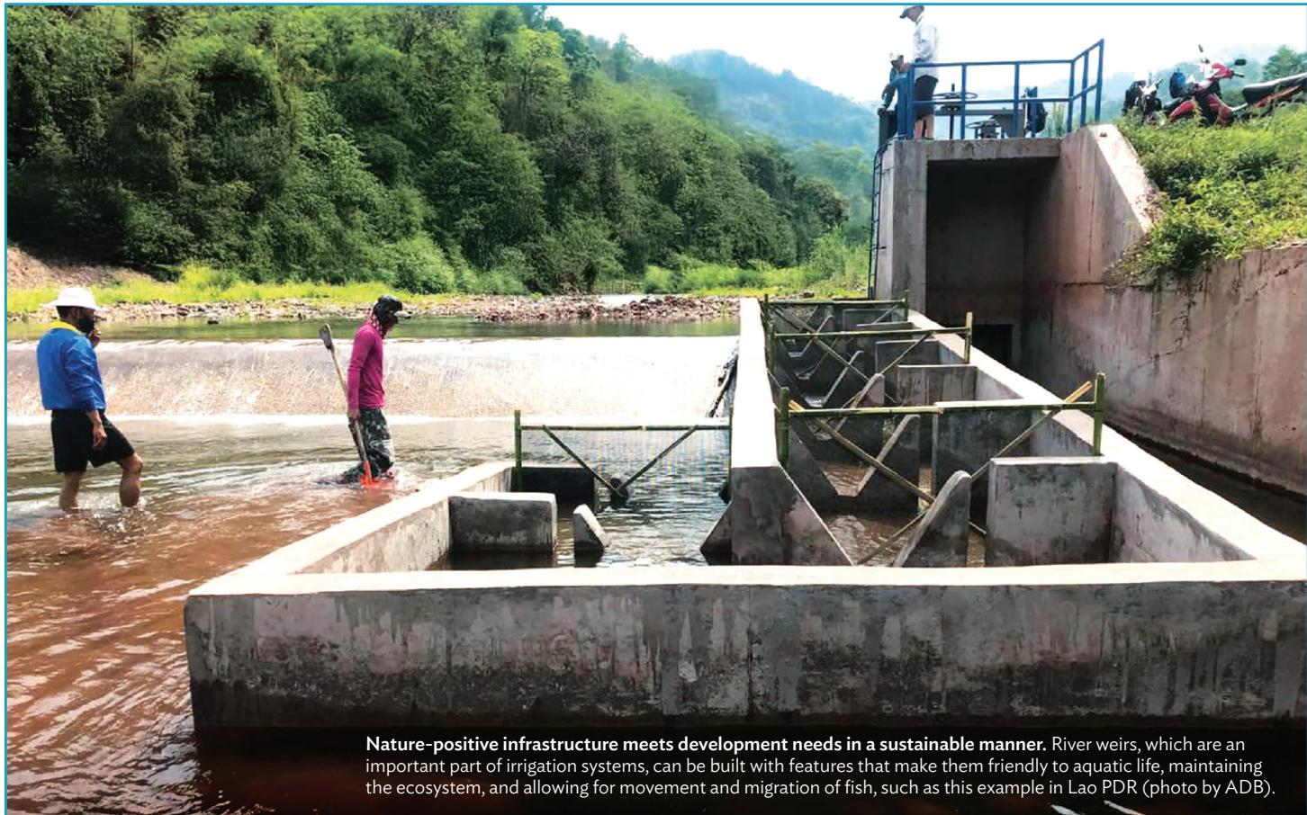
**Nature-positive infrastructure meets development needs in a sustainable manner.** River weirs, which are an important part of irrigation systems, can be built with features that make them friendly to aquatic life, maintaining the ecosystem, and allowing for movement and migration of fish, such as this example in Lao PDR (photo by ADB).
