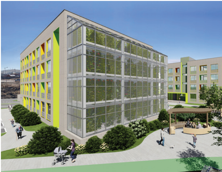
Building A – Multi-story greenhouse
