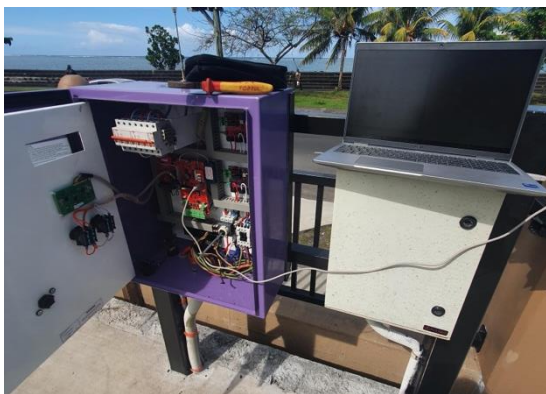
Installing telemetry units for remote monitoring Source: Samoa Water Authority
