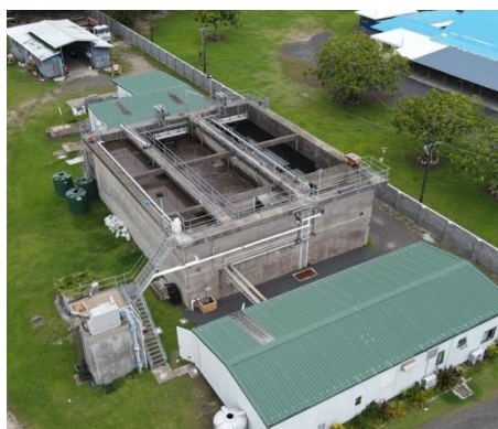
Wastewater Treatment Plant, Sogi, Apia Source: Samoa Water Authority
