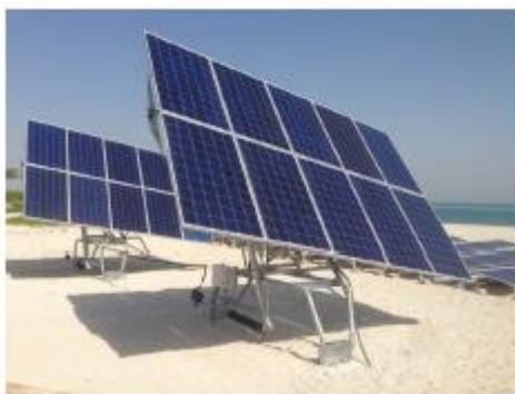
Figure 27: Helioslite 1.5 tracking system
