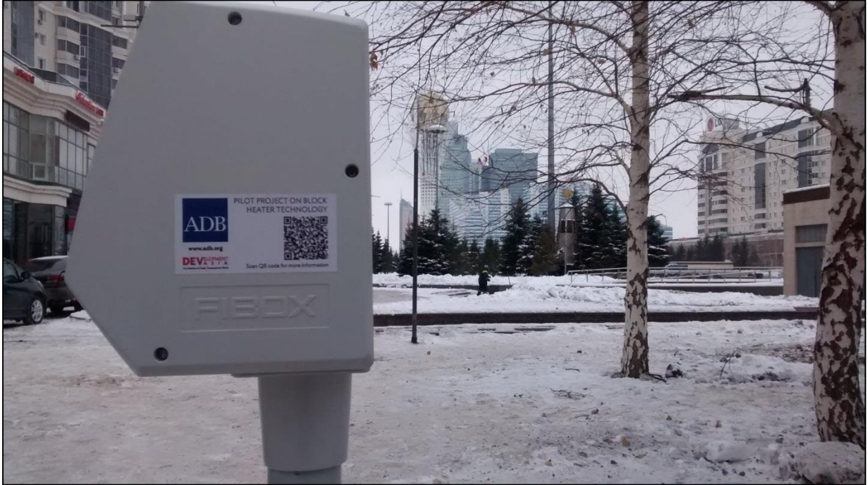
Exhibit 21 QR Code on Charging Pile Station for Public Awareness
