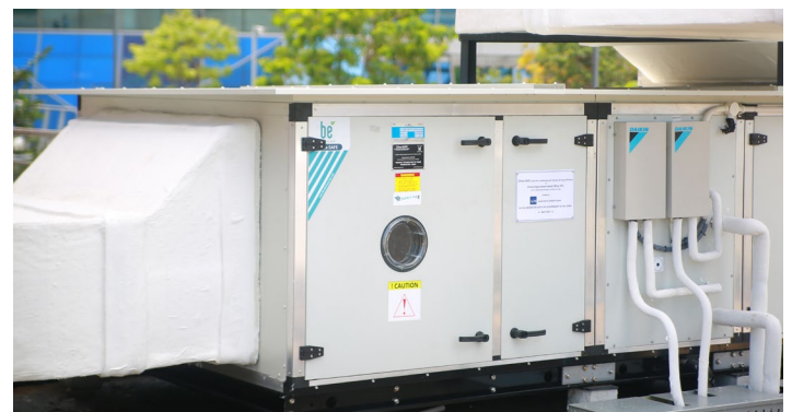
Smart air handling unit with filtration and efficient cooling units
