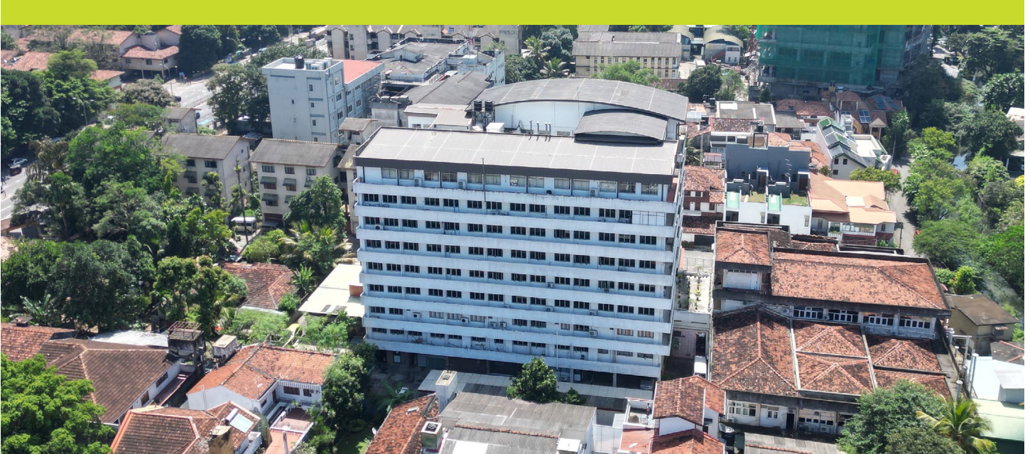
Aerial view of the Sri Lanka Standards Institution building
