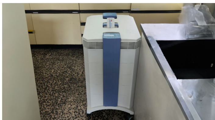
Portable filtration system to improve indoor air quality
