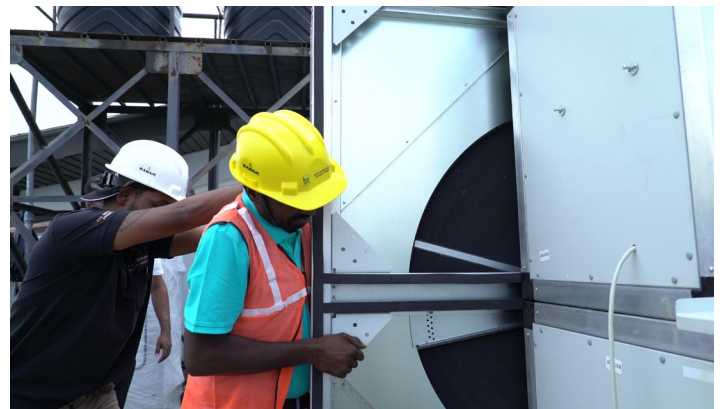
Installation of heat recovery wheel
