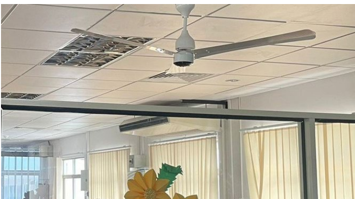
Energy-efficient and silent ceiling fan with brushless direct current motor and remote control
