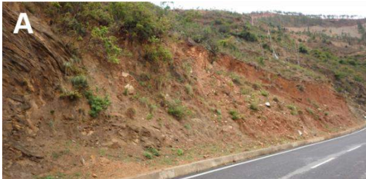
A: Slope before vegetation works on May 29, 2019
