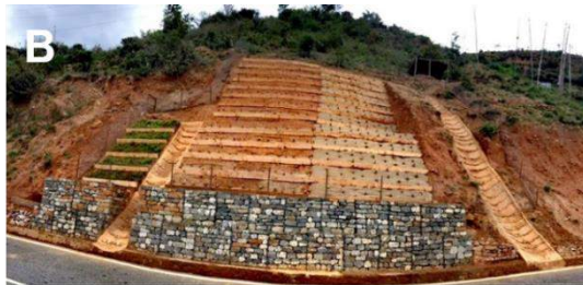
B: Finished vegetation works on May 30, 2020
