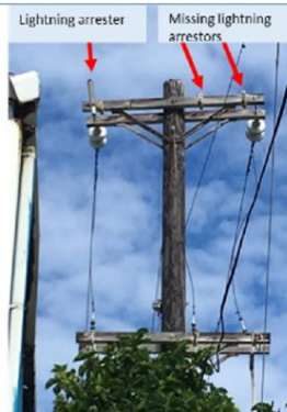
Lightning arrester
