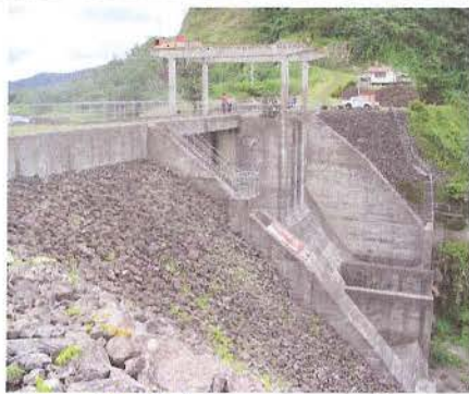
Figure 12: Hydro power provides about 50-60% of electricity generation. Mini hydro potential sites will be explored and assessed.
