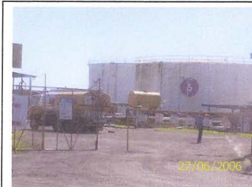
Figure 15: Petroleum storage facilities must adhere to national and international safety and quality standards.
