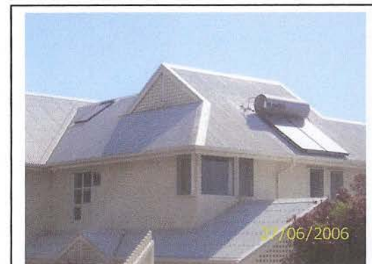
Figure 10: Solar water heaters are widely used in hotels and private homes and other small businesses
