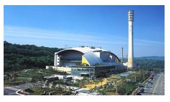
The facility was created in May 2005 after prolonged use of landfills for the northwest region of Seoul. It has the capacity of incineration for 750 tons of waste per day (250 tons per day × 3 units). The wastes are safely incinerated at high temperatures. Recycled
